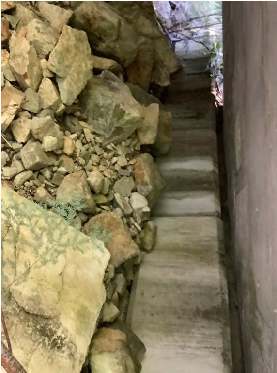
Right Bank Abutment when facing downstream
