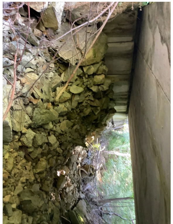
Left Bank Abutment when facing downstream
